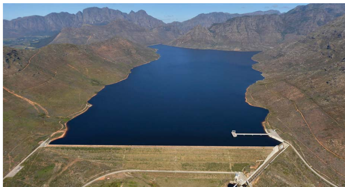
A dam fine sight: The Berg River dam was almost full last week, and overall, the dams that supply Cape Town were 76% full.
