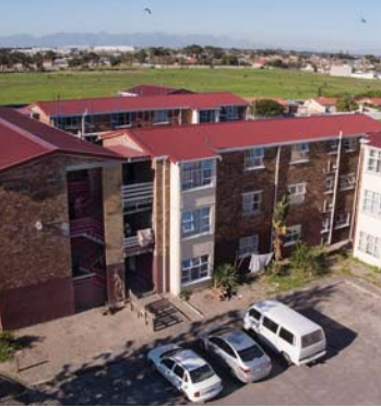
Aylesbury Court in Ottery before a R7,2 million upgrade.
